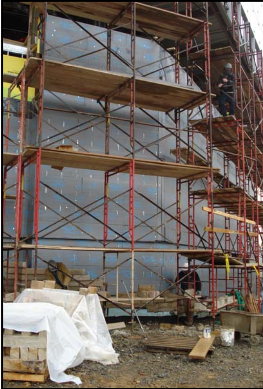
Figure 11: Masonry work on the East end of the building around the auditorium.
