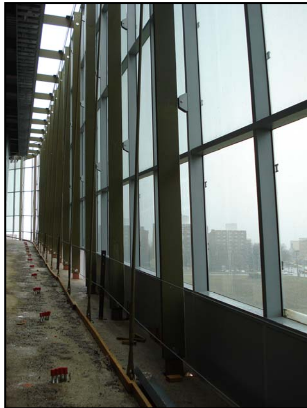
Figure 23: Image from inside of the building at CW-4 showing steel strong backs at study carrels.
