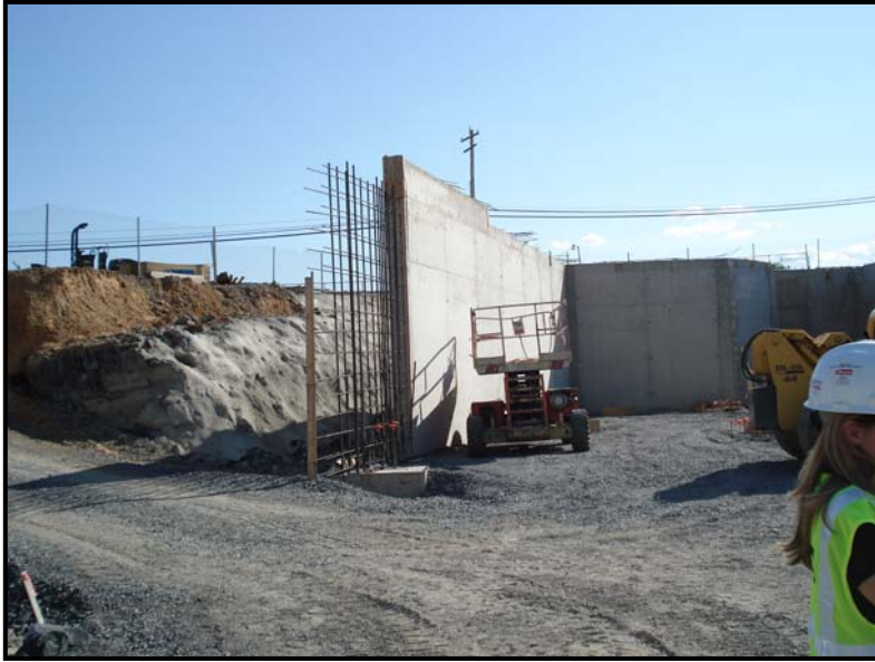
Figure 9: Image showing construction ramp, rebar reinforcing for walls to be poured, and some of the poured walls on the west end of the building.
