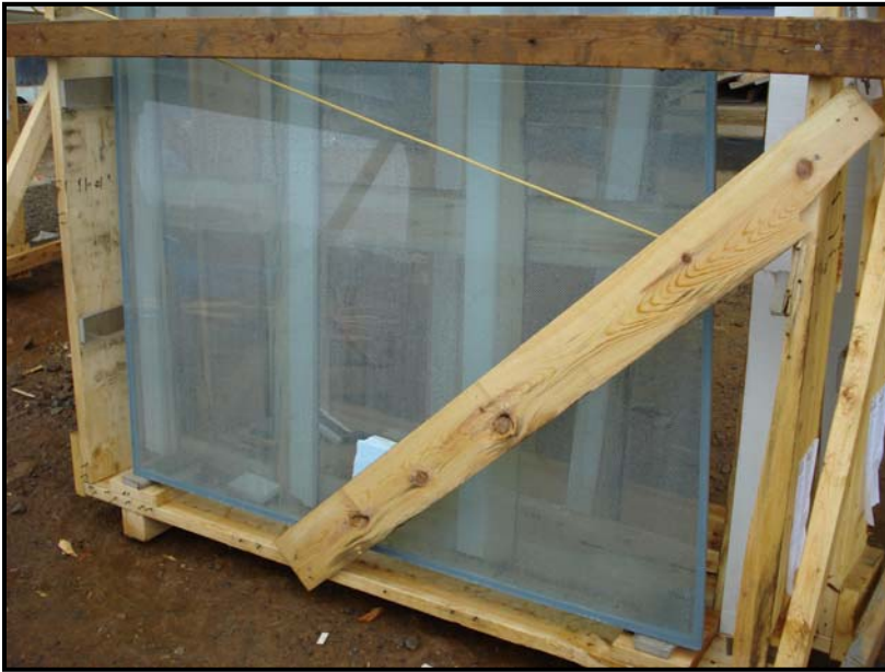
Figure 21: Double pane glazing being stored onsite until workers are ready to install it in the curtain wall.
