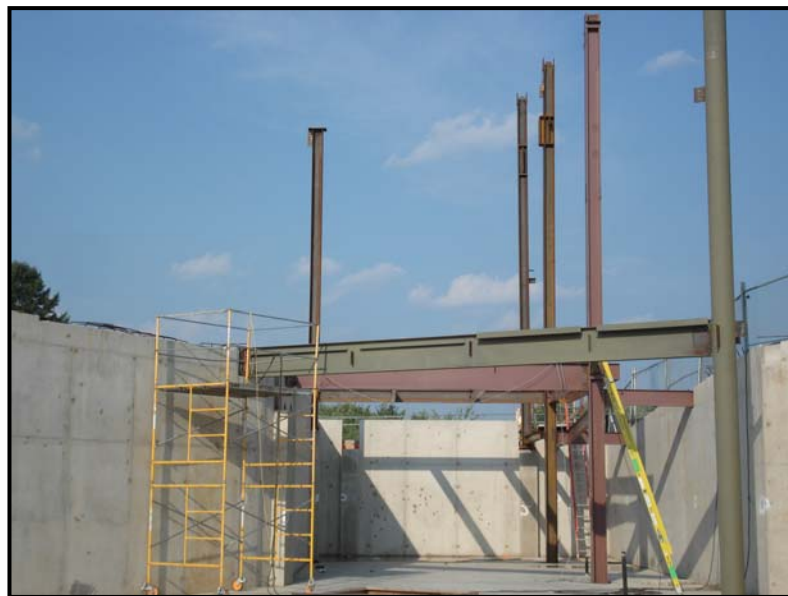
Figure 10: Image showing steel erection progress on the East end of the building early in the erection phase.
