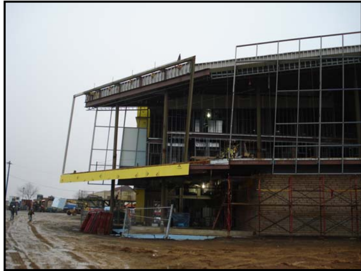
Figure 5: Masonry and Curtain Wall Framing on the South Side of the Building.
