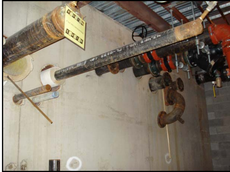
Figure 12: The campus utilities entering the building.
