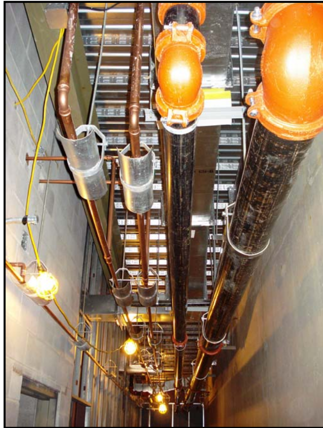
Figure 15: Image of the corridor plenum space in the lower level of the building.
