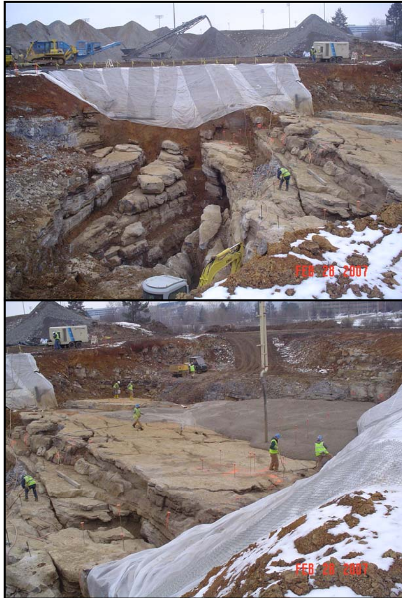
Figure 8: A view of the large sinkhole that ran underneath the building footprint (top) and a view of the process of filling the sinkhole with concrete.
