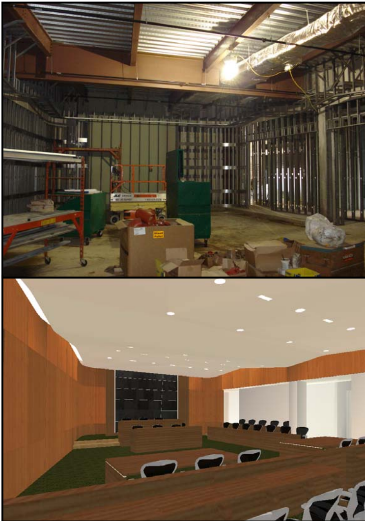
Figure 7: A view of the courtroom construction (top) and the same view of a rendered virtual mockup of the courtroom. (bottom)
